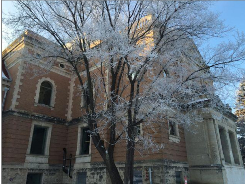
Figure 12. Taché Arts Complex (exterior of Music Library)
